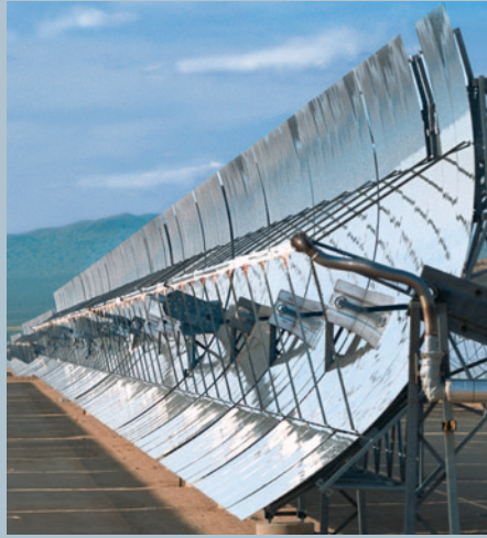
聚光式弧型集熱槽 (Parabolic trough)
